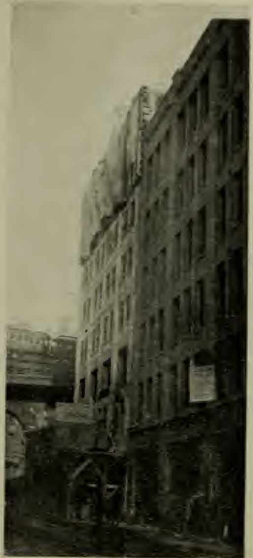
FIG. 7. UPPER STORIES ENCLOSED WITH TARPULINS.
